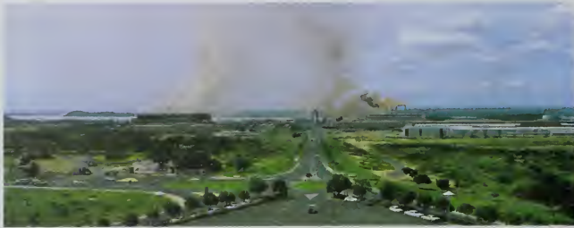
Steel mill at Matanzas, part of the major industrial centre of Ciudad Guayana at the Orinoco-Caroni river junction.
